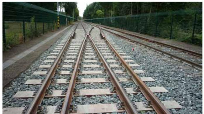
The ecological compatibility of the polyurethane ties is also an advantage. As a rule, ties that have already been in service can be reused, or can be recycled in the same way as the production scrap.
