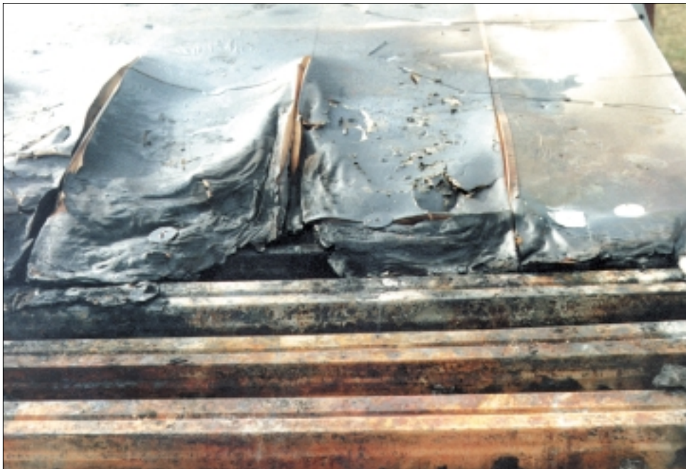
Figure 8: Roof after test - Pentane blown foam
