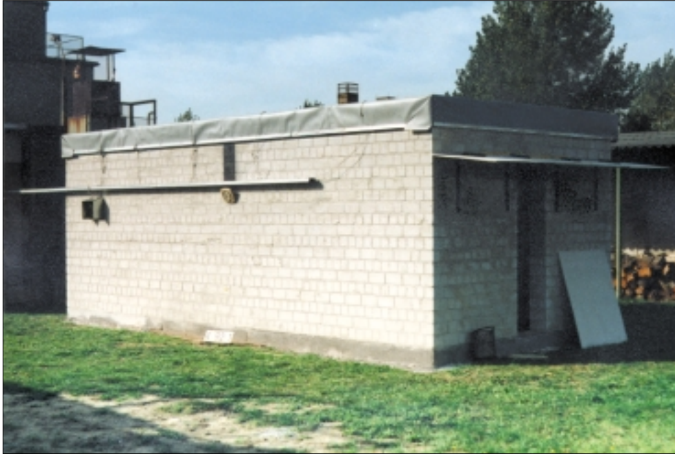
Figure 1: Test building at Leipzig
